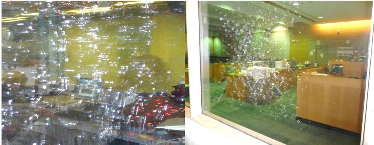
This CGJ found security windows cracked, some with heavy spider web cracks.
