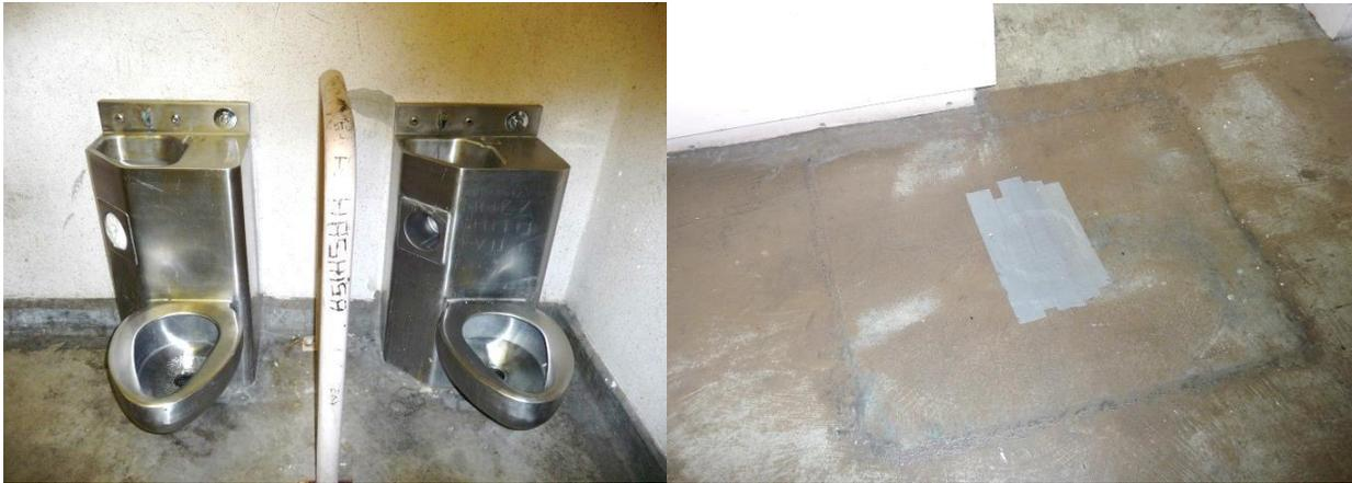
Plumbing and sewage issues are a problem with inoperable toilets and sinks. Jailers have to find ways to control the odors (such as taping over floor drains).
