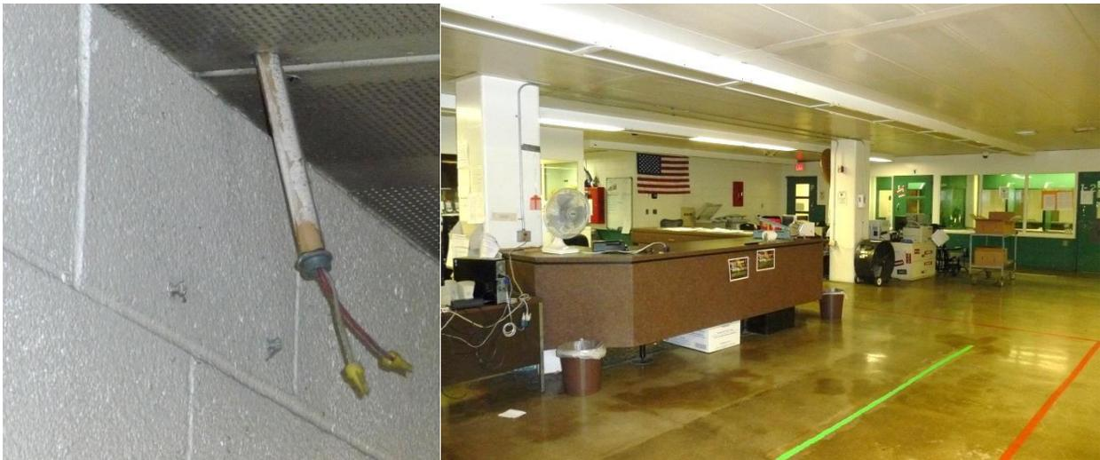
This CGJ found exposed electrical wiring. The deputy we talked with speculated that it had initially been designed to accommodate emergency lighting. The deputy noted that there is only one emergency light for the detention area and the power is interrupted about once a week. To address this, the deputy sheriffs all carry flashlights on their belts.
