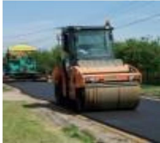
Steam Roller is the most efficient and complex way to repair potholes. This involves complete resurfacing of the street. <http://thenewswheel.com/5-kinds-pothole-repair>
