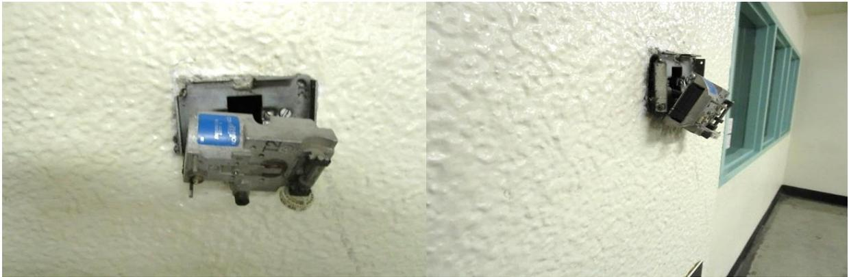
There is a climate control box on the 8th floor that is hanging off the wall. It apparently had been damaged for quite a while.
